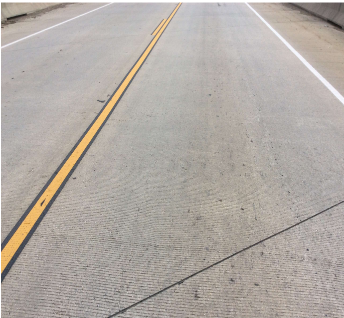
PHOTO 1 Description Deck - Span 2 right (longitudinal cracking)
